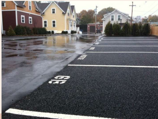
Cottages on Green, East Greenwich, RI Photos courtesy of Jonathan Ford, Horsley Witten Group
