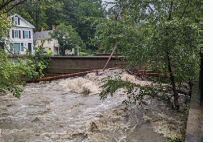
The North Street Bridge was not designed to accommodate current flooding. As a result, the bridge acts like a dam. The river backs up behind the bridge, overtops its banks and floods downtown Williamsburg.
