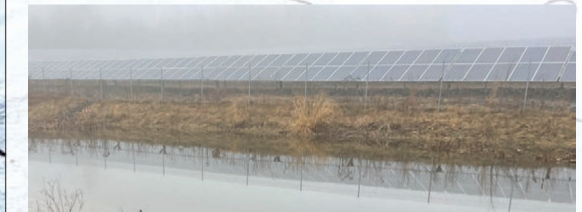
Runoff from a large ground-mounted solar facility in Williamsburg had devastating impacts to the West Branch Mill River and local wetlands and required extensive remediation.
